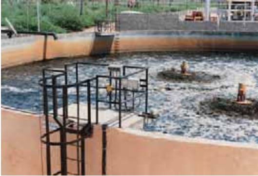
Common effluent treatment plant for industrial park
