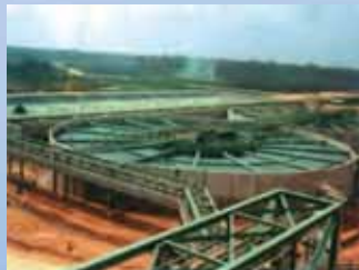
High rate solids contact clarifier
