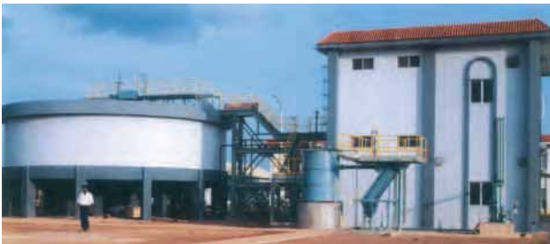
Sludge handling system
